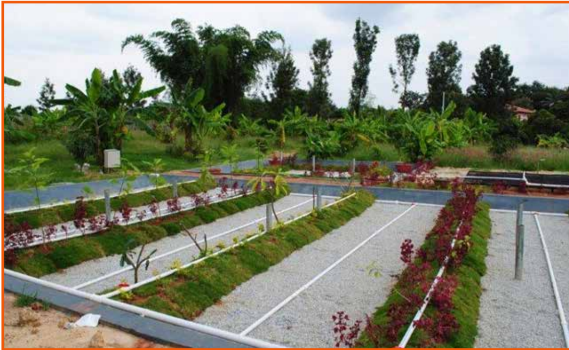
Figure 16: Bioreactor 1 (BR1) in the foreground with Bioreactor 2 (BR2) and treated water tank in the background
