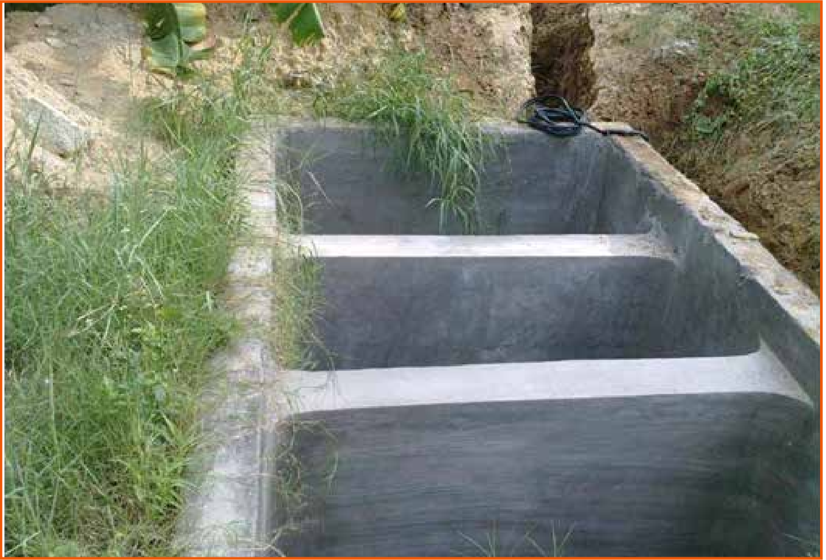
Figure 14: Septic tank extension compartments
