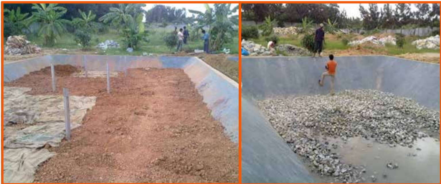
Figure 13: Construction progress, bioreactor walls lined, and media being filled into BR1
