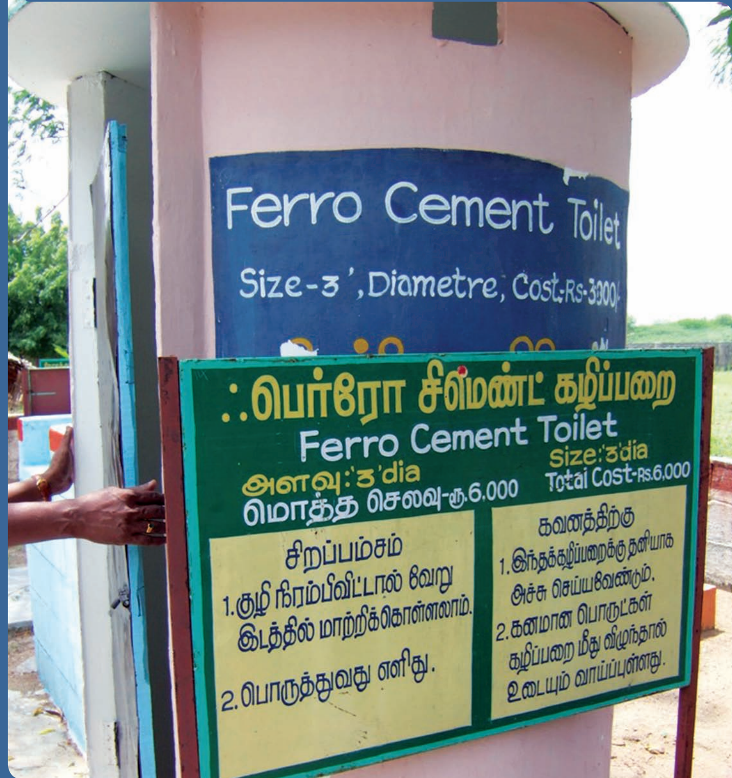
IMAGE 10: Low cost ferrocement superstructure: Gramalaya
