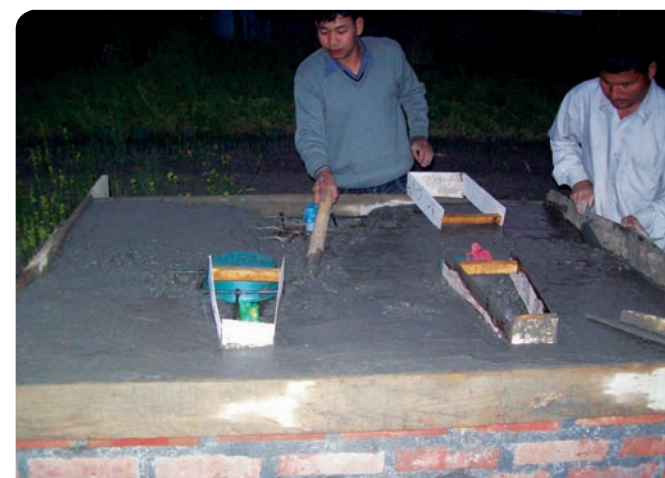
Step 5: Pans fitted over the chambers
