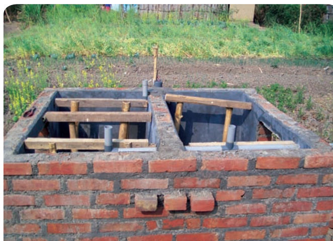
Step 4: Ready to be fitted with the slab
